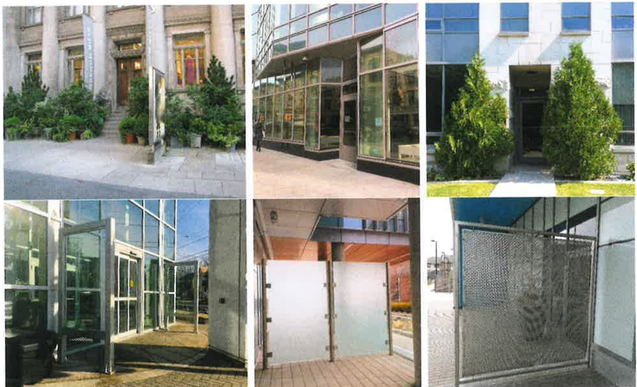
Image 7: Examples of Wind Control Measures Applicable to the West Entrance of Building 1
